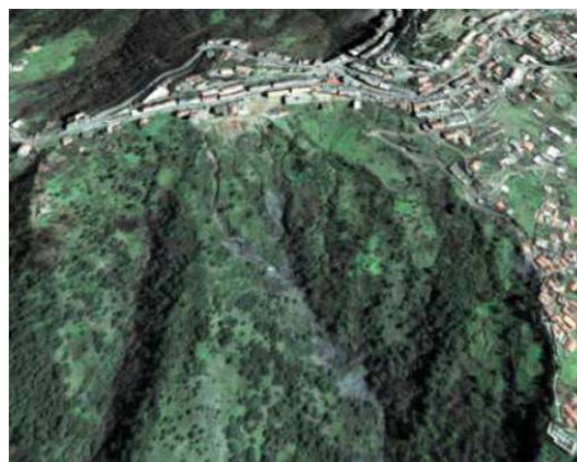
Fig. 1 Satellite view of the location of AEH landslide
