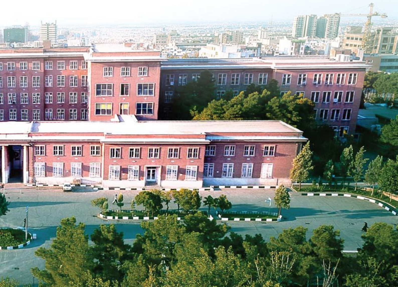
Imam Khomeini Hospital Complex
